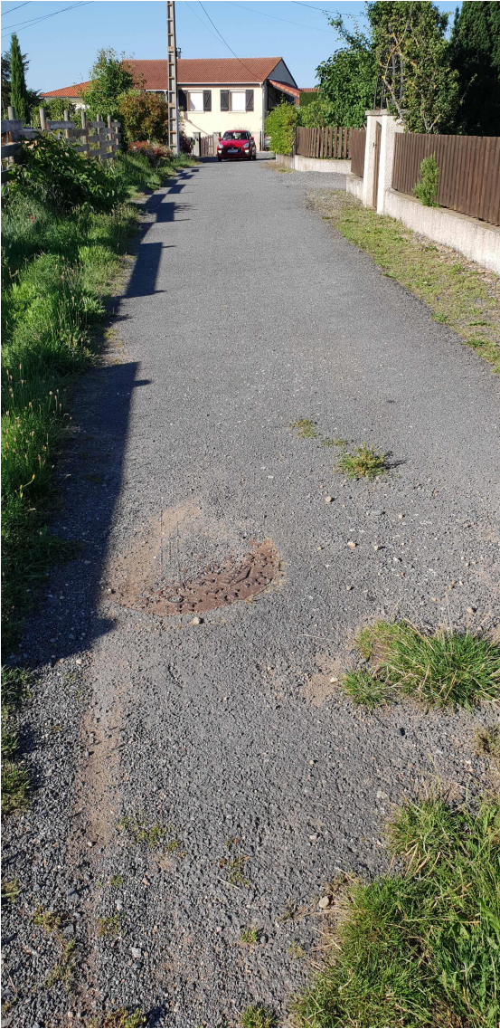
PHOTO 3 EGOUT DE BRANCHEMENT
